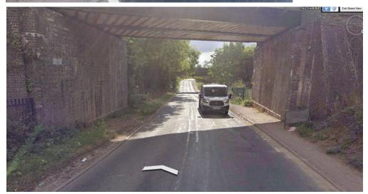
Appears to be sufficient width to re-locate motor-vehicle lanes approx 1 metre to the left and create a ≈2m wide shared use path.
