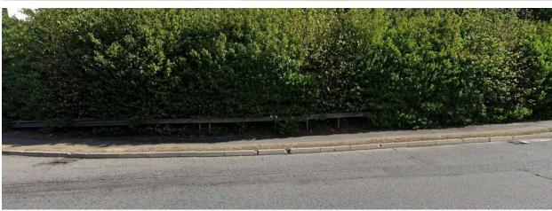
Also at this location, completely inadequate and poorly maintained pavement width, this is not even adequate for a single pedestrian, let alone for a bidirectional shared use path. Needs to be at least 3m wide.
