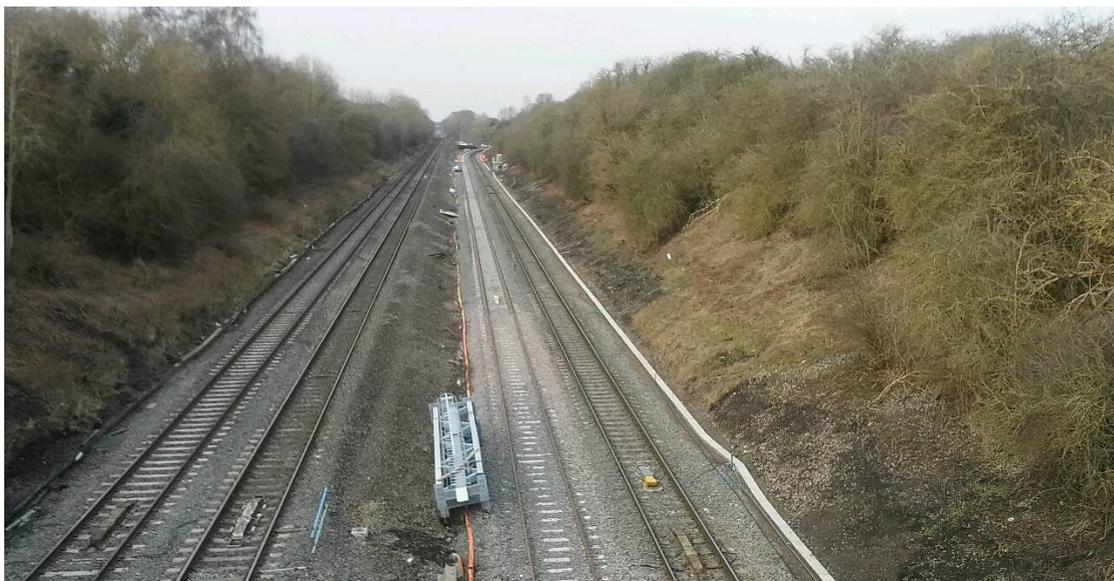
*The Midland main line between Bedford and Kettering where a fourth track has been reinstated and electrification masts are ready to be installed*
